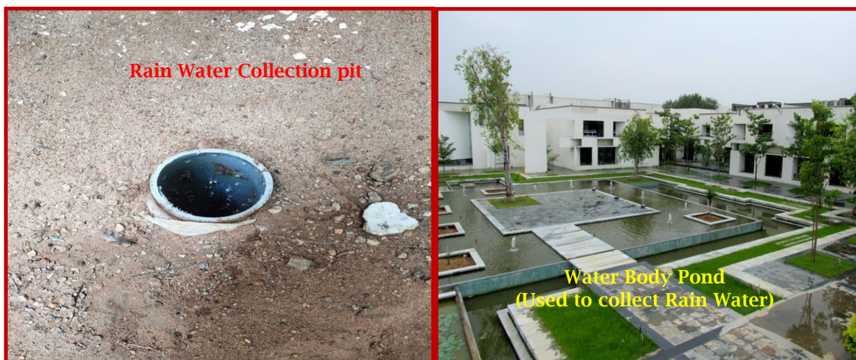
Fig.5: Rain Water Harvesting (RWH) system implemented in the College
