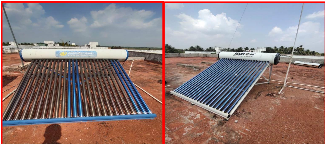
Fig.7: Solar Thermal Hot Water Generating System for Bathing Application
