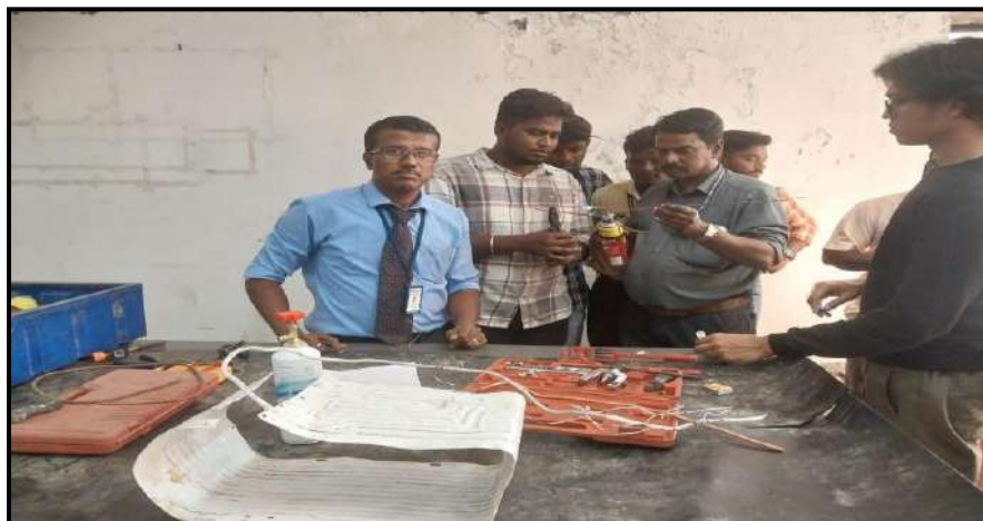
Practical Demonstration of Brazing of Copper tubes
