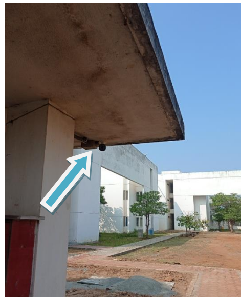
CCTV Camera Installed at Girls Hostel Entrance
