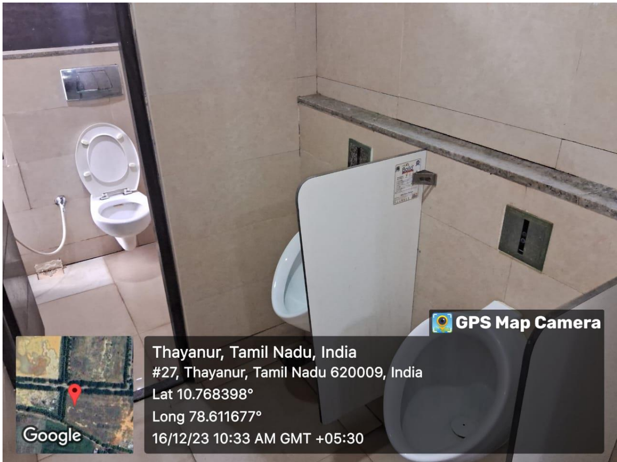
Fig. 7.1.2.3 Sensor based Urinals.
